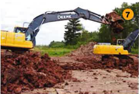
7 Backfill excavation and cleanup
