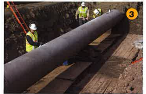
3 Clean the exposed pipe
