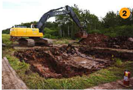
2 Excavate to expose the pipe
