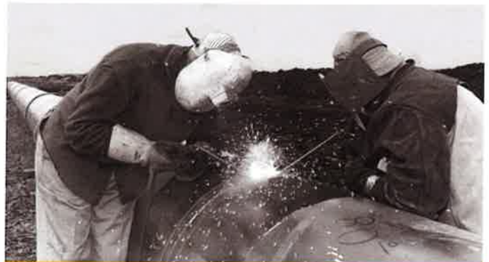
Enbridge Mainline pipeline construction from the 1960s.
