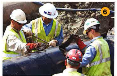
6 Re-coat the pipe
