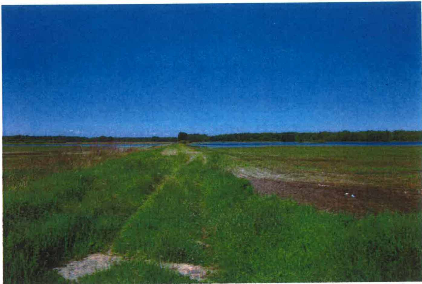
Far East End County Ditch 24 Looking West on 6/25/2012 During Flood Conditions
