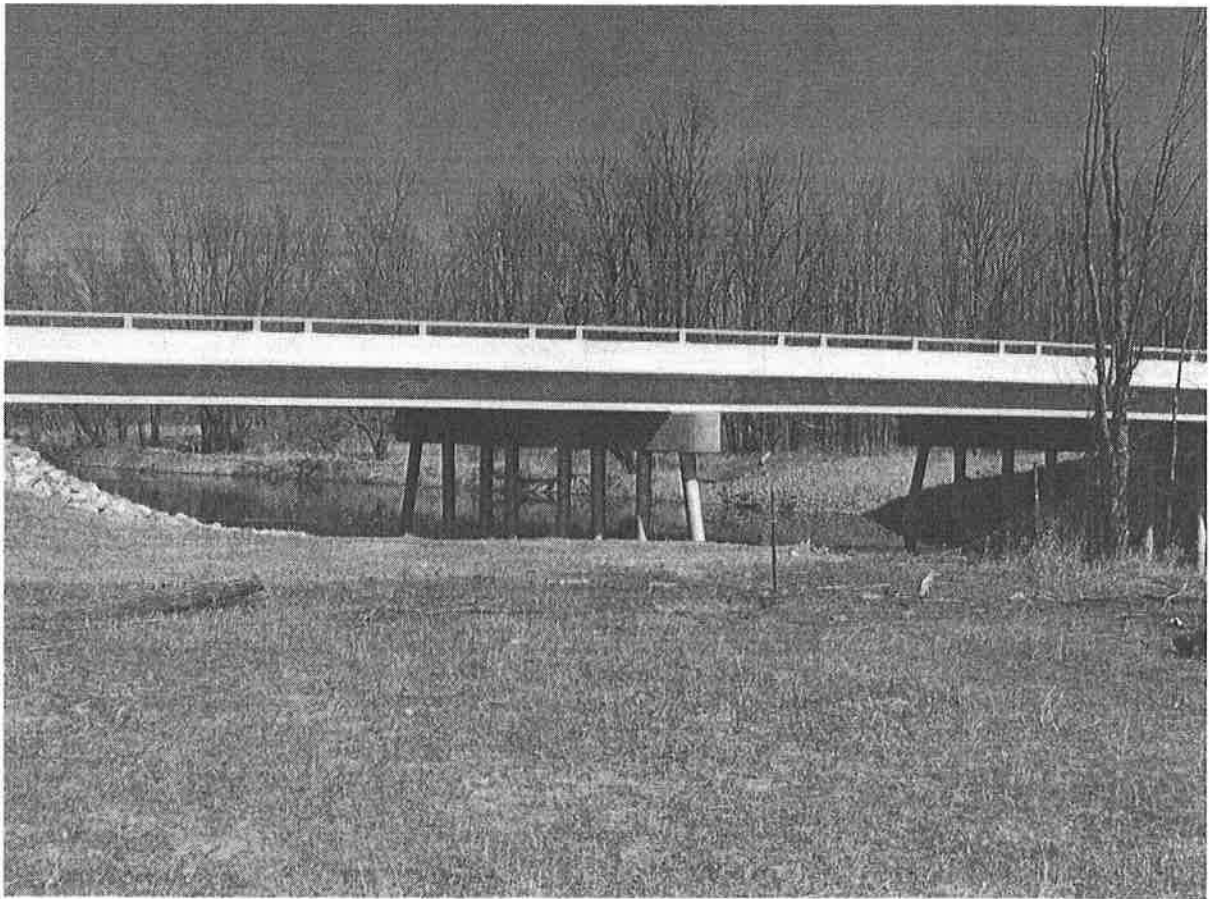
County State-Aid Highway 3 Bridge over Willow River
